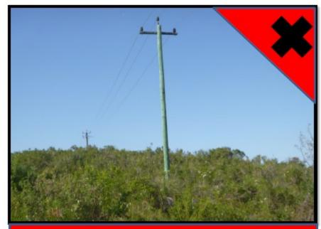
Thick scrub around the base of a power pole creates a potential fire hazard
